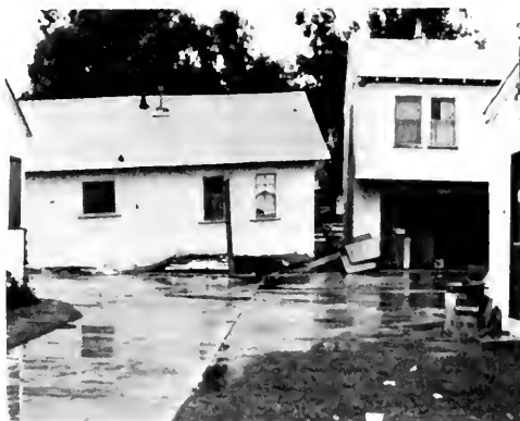
Photo 4. Wood frame structure in center was two stories high; note automobile beneath.
